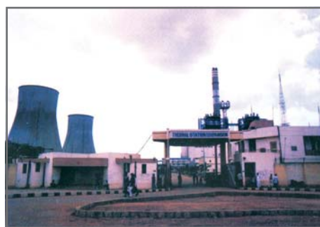
Fig 3.12: A view of a Thermal Power Station
