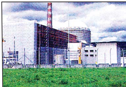
Fig. 3.18 : Nuclear power station , Kalpakkam
